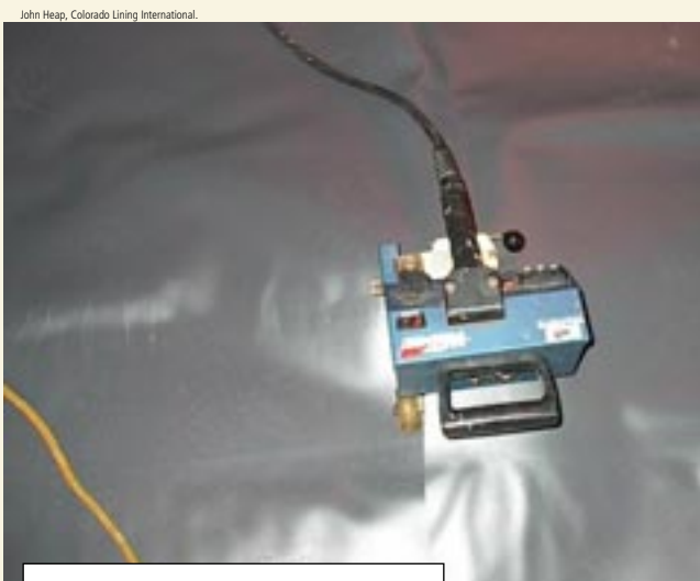
Photo 1b. Hot-wedge welding.
